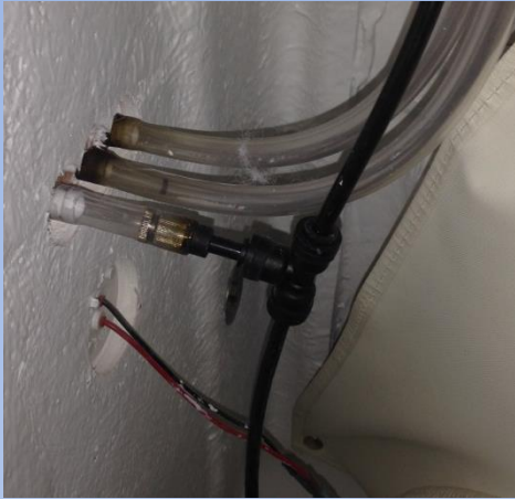
Typical Automatic Drain Valve (ADV) installation
